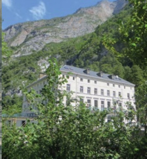
Station Thermale des Eaux-Chaudes.
